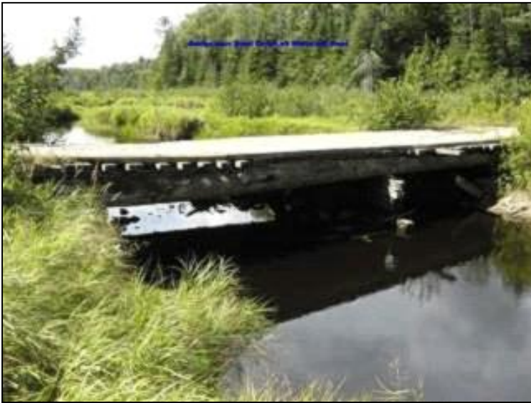
Bridge on Gold Mine Trail (C8) in Parishville
