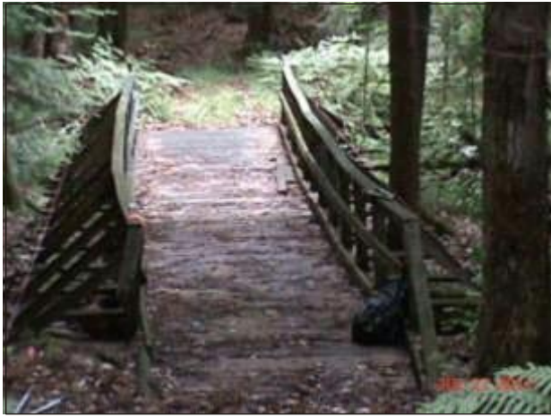
6' wide bridge Clear Pond (C8) in Parishville.
