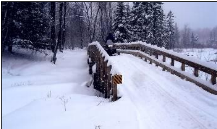
Middle Branch Bridge – Stillwater DEC labor and our material
