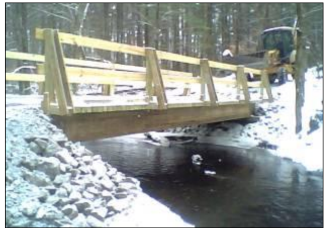
New bridge at the CC Dam in Brasher State Forest – Glu Lam Beams from Wanakena
